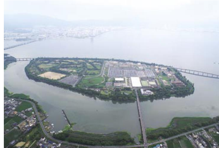
Konan Central Treatment Plant
