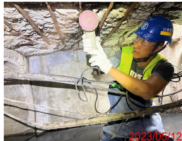
TYPE A 局部頂板鋼筋鏽蝕
